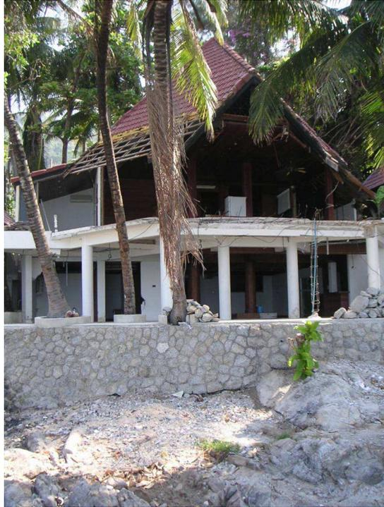
Figure 6.10: Picture taken in Patong Beach in Thailand showing the run-up ramped into second floor.
