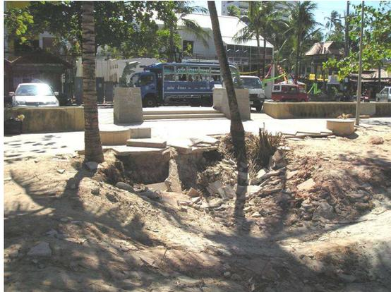
Figure 6.23: The picture was taken from [Dalrymple and Kriebel, 2005] and it shows a pedestrian seawall opening correlated with damage. The most important damage appears in front of the opening.
